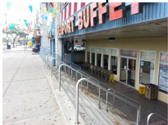
Below grade retail space in cellar
