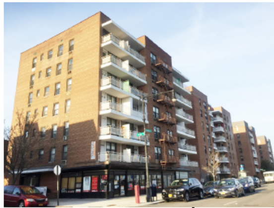
Seven-story apartment building on eastern end
