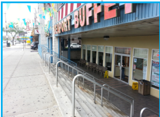
Below grade retail space in cellar
