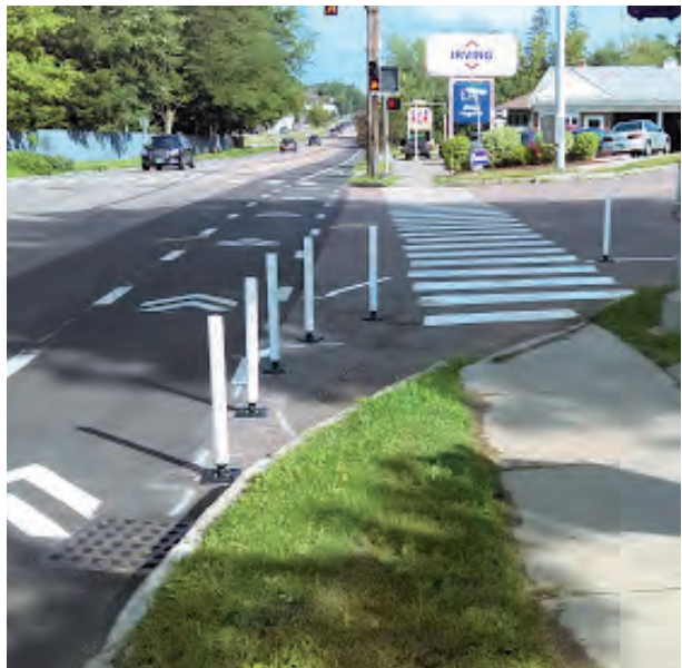
Figure 2.13 Flexible delineator posts near a pedestrian crossing. Source: Tactical Urbanist’s Guide.
