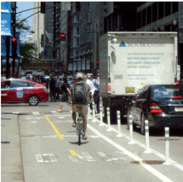
Figure 2.8 Two-way separated bike lane. Source: Chicago Department of Transportation.
