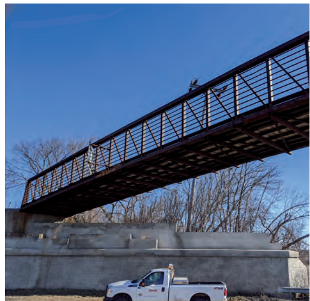
Figure 2.19 Robert McClory trail with significant vertical clearance over IL 173 in Zion. Source: Google.
