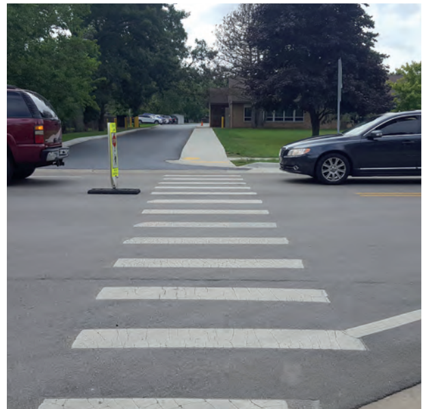
2.15 Marked crosswalk with in-road Must Stop for Pedestrian sign on 9th Street at Russell Avenue near Westfield School in Winthrop Harbor.
