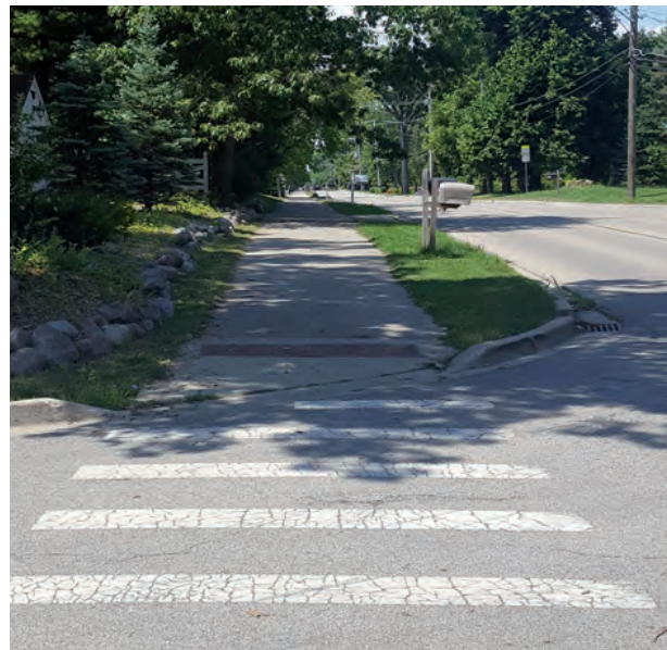
Figure 2.17 Sidepath on Wadsworth Road in Beach Park
