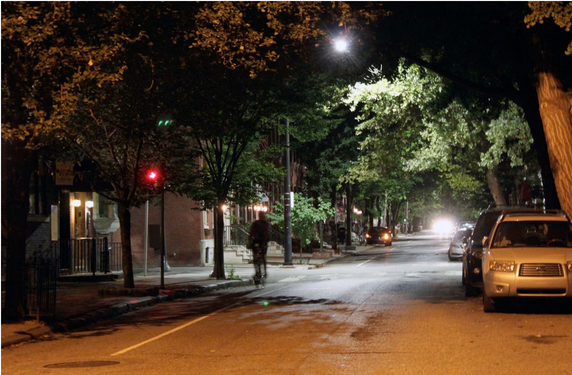
LED lighting in the background vs high pressure sodium lighting in the foreground on Spruce Street. In addition to considerable energy savings, LED lighting better illuminates roadways for pedestrians, bikers, and drivers.
