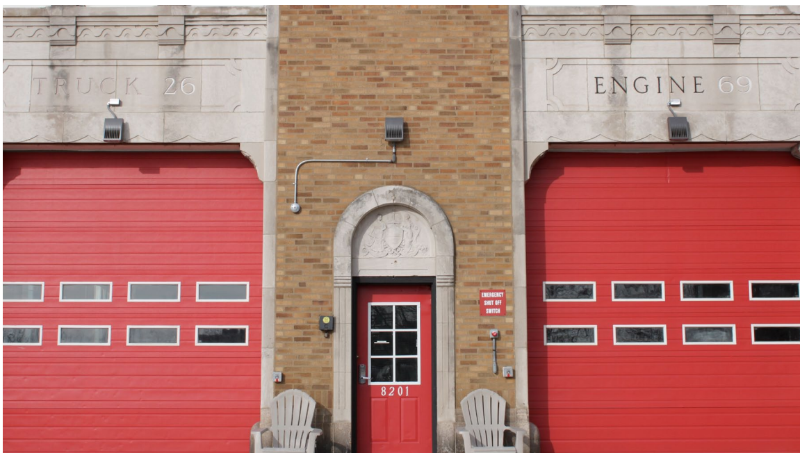
Through the EESF, the City has installed LED lighting in many City facilities, including Fire Engine 69, shown here.
