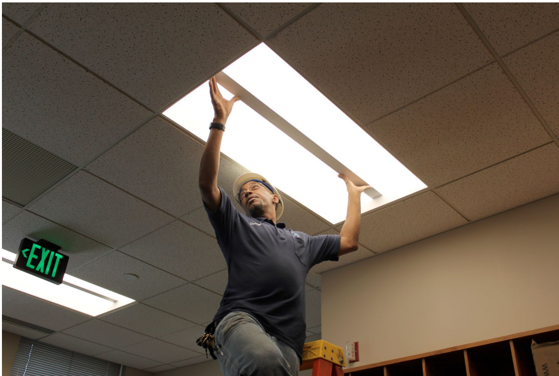
Operations and maintenance personnel installing LED lighting at One Parkway Building.
