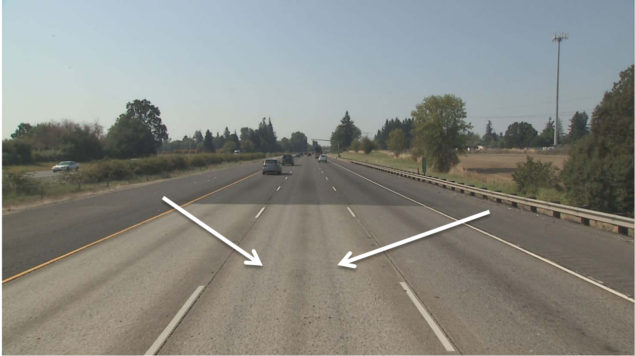
Figure 4.3: Studded Tire Ruts
