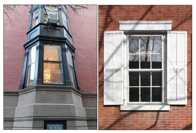
**Criteria:** Exterior storm windows should have tightly fit framing within the window openings without the need for a sub frame or panning around the perimeter, with meeting rails used only in conjunction with double-hung windows.
