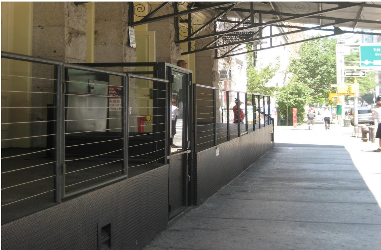
Figure 6 A platform lift with clear glass finished to match the adjacent building finishes.
