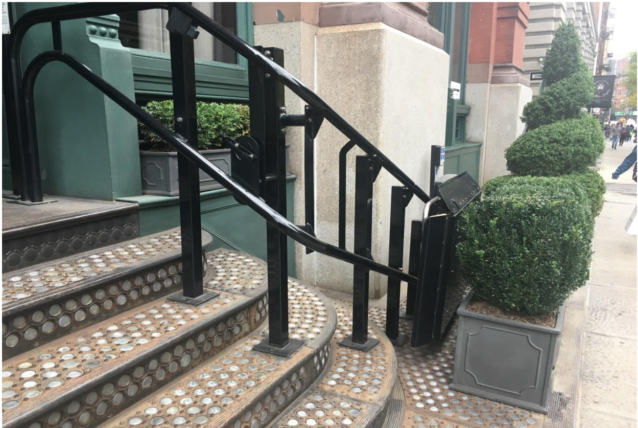
Figure 4 A mechanical lift finished to match the surrounding materials and therefore recede from view.
