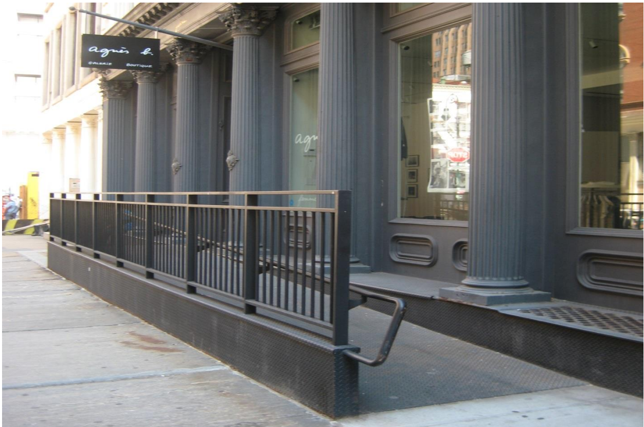
Figure 2 A simply-designed ramp with steps and handrails.
