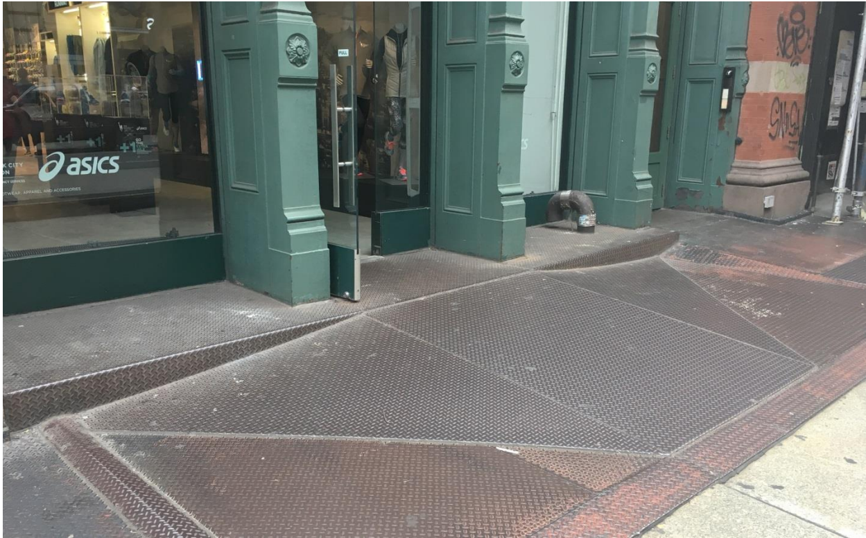
Figure 3 A ramp that harmonizes with the existing features and materials of the building.
