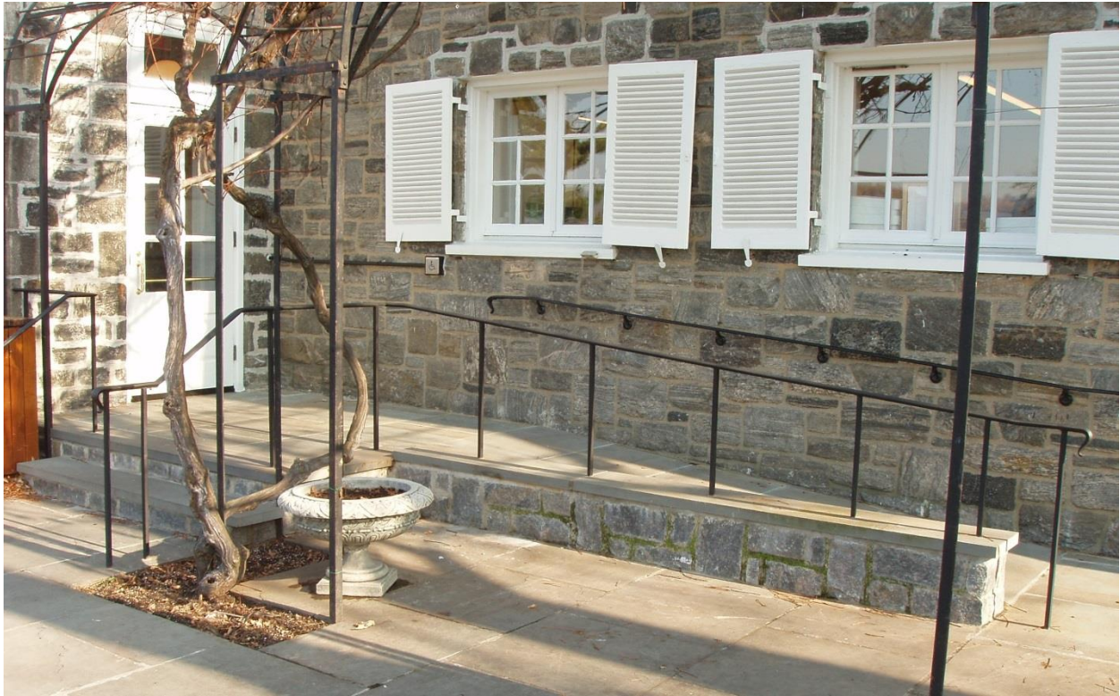
Figure 1 A ramp installed at a primary entrance with materials matching the historic building.
