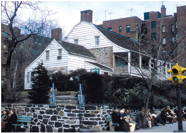
The historical context section should note if a project contains a designated New York City landmark, such as the Dyckman Farmhouse. Photograph by LPC.
