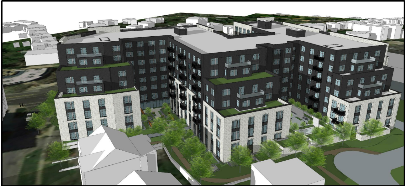
Figure 6 – Perspective of Building’s rear setback and stepbacks from residential neighborhood looking towards Old Georgetown Road
