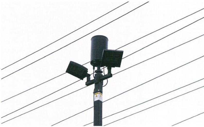
Existing small cell antenna in Rockville. Source: Bethesda Magazine.
