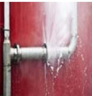
EXCESSIVE LEAKS
