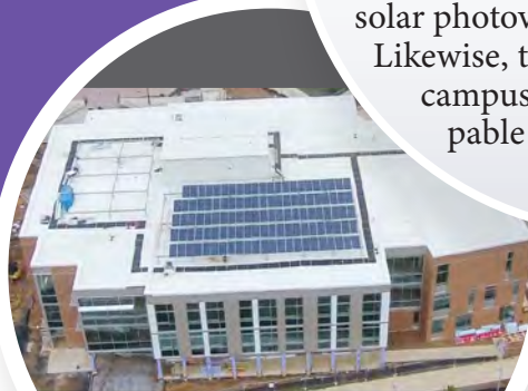
Rockville Campus Science West Photovoltaic Array
