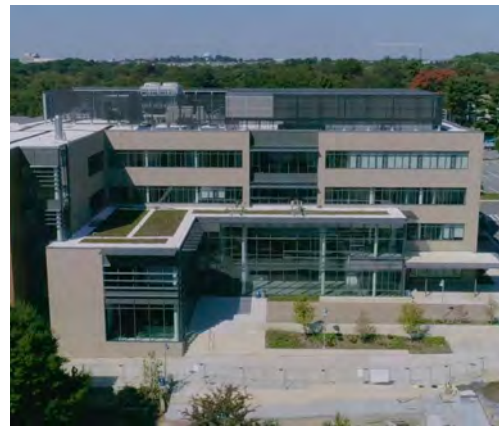
Long Nguyen Kimmy Doung Student Services Rockville Campus Opening July 2020 LEED Gold Targeted
