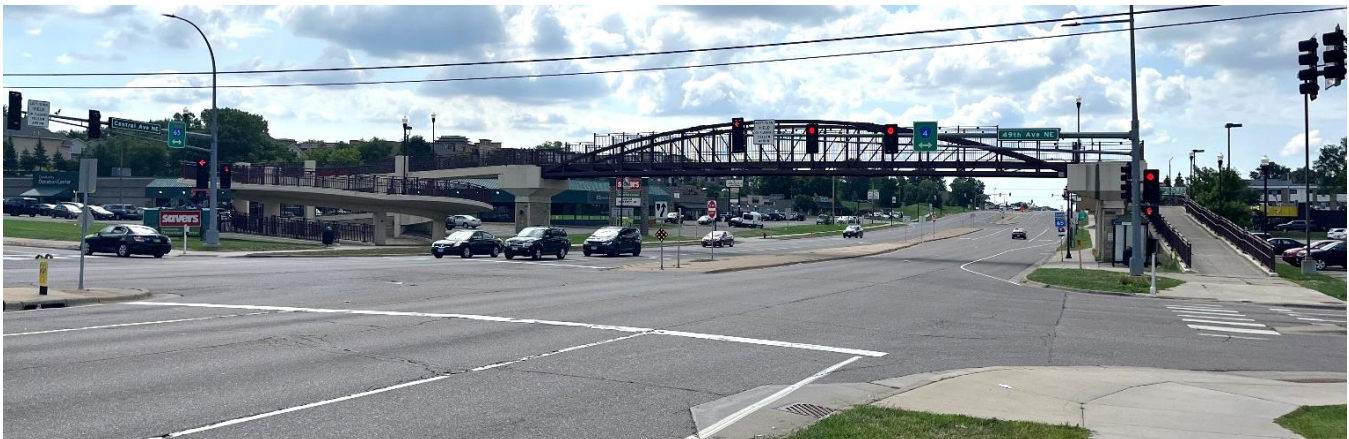
View south down Central Avenue at pedestrian bridge and proposed platform locations (Source: Metro Transit)
