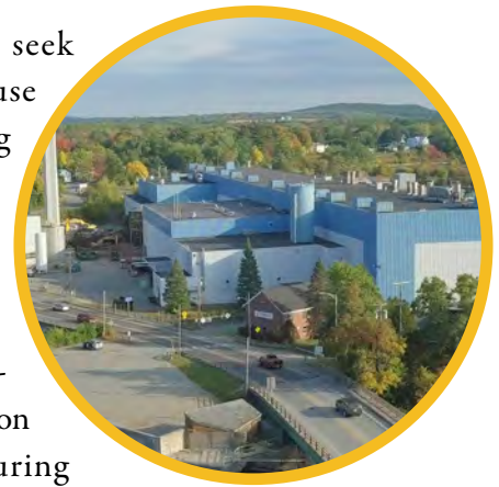
Maine-based startup GoLab is expected to start making climate-friendly wood-fiber insulation in this former Madison paper mill in 2021.
