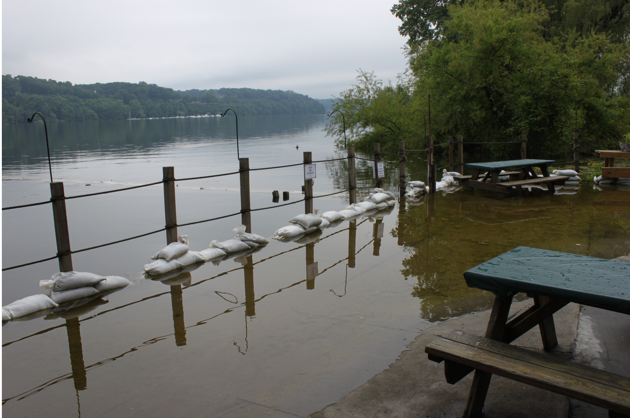
Pictured above, flooding of Sandbar Park in the town of Webster, Monroe County, in 2019.
