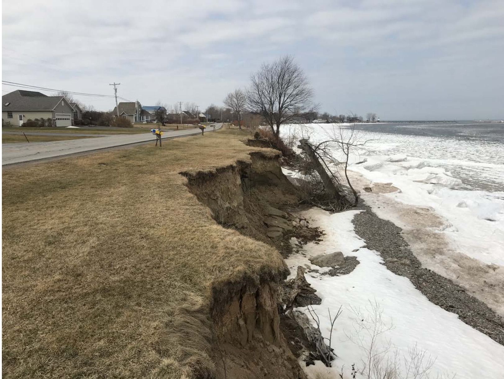
Pictured above, erosion of original Lakeside Park Road West access road, in the town of Carlton. The road was degraded due to repeated flooding events.
