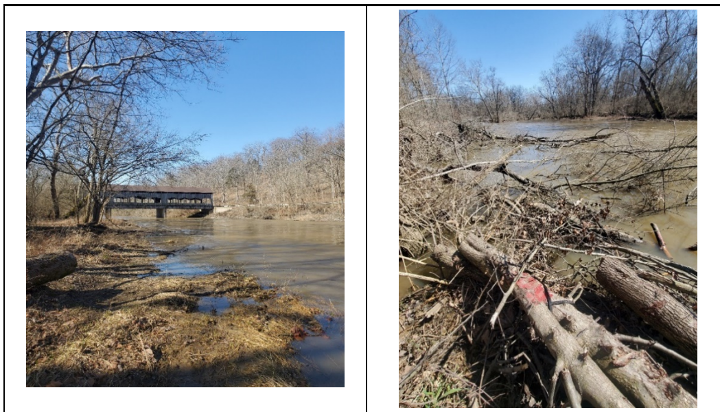
Left: Upstream of Installation; Right: Upstream view with Flow Kicker
