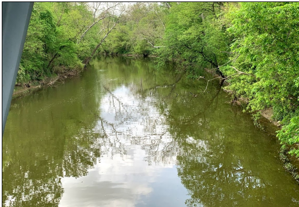
Location: Stillwater River, Barnes Road, Webster Township, Darke County. Installation completed over 20 years ago. Photo Source: Elizabeth Myers, OU, May 2021
