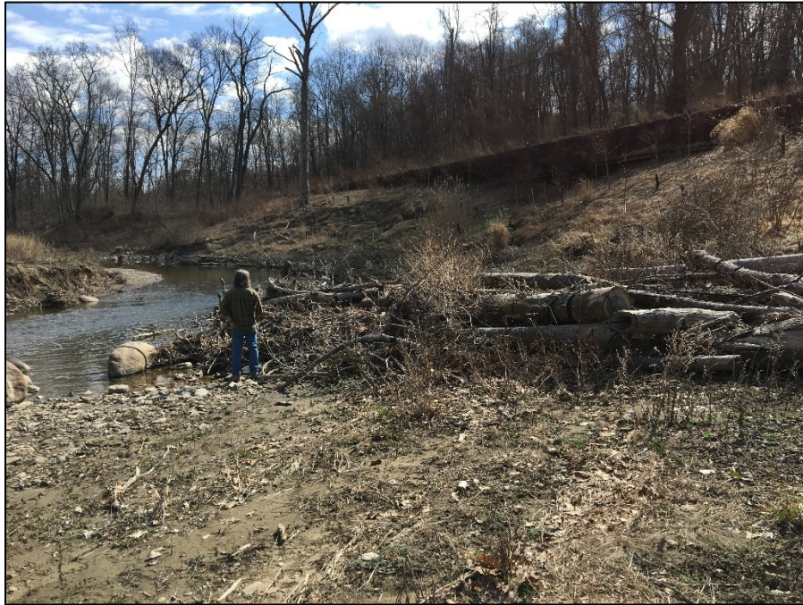
Installation of Flow Kickers Shown. Photo Source: Karel Cubick, MS Consultants, March 2021 Figure 14: Yellow Creek Installation, Facing Downstream
