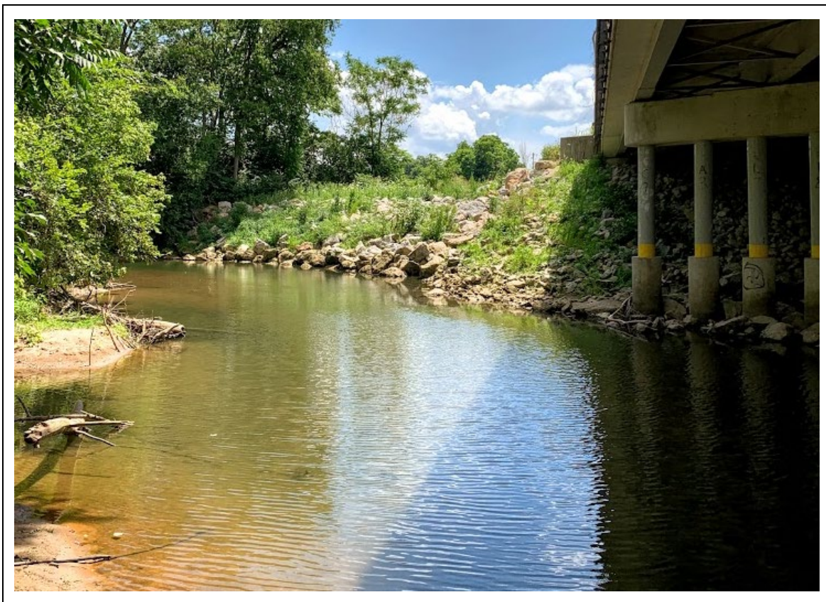
Figure 9: Riprap Applied for Bank Stabilization
