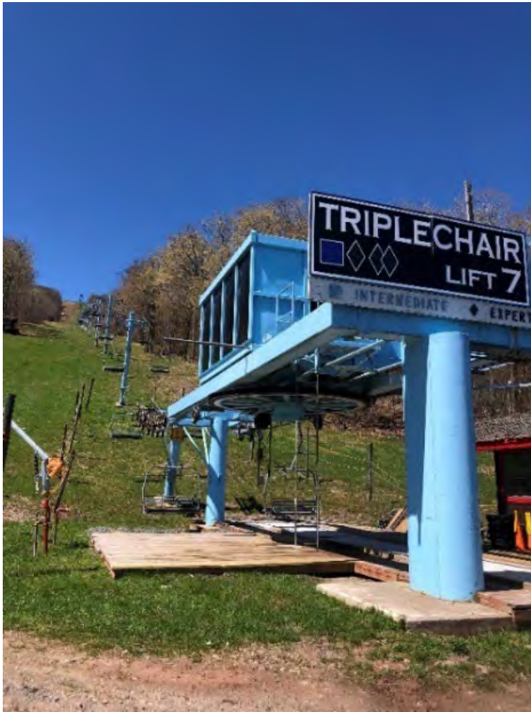
Image 1 : Existing Base of Lift 7
