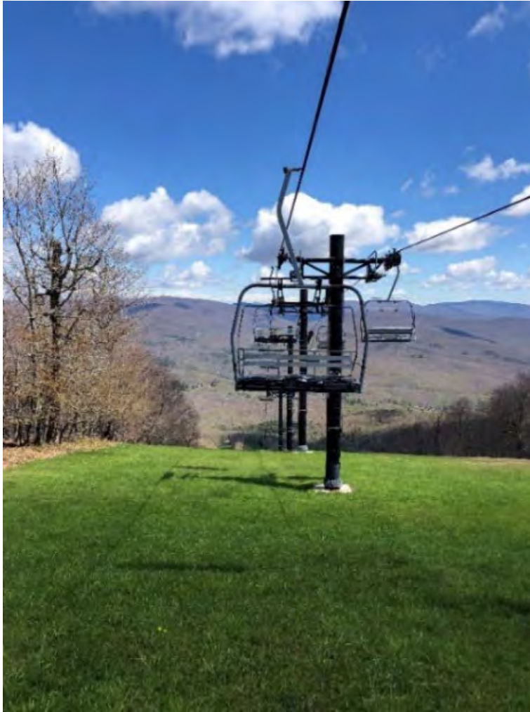
Image 2: Existing Top of Lift 7
