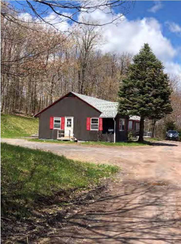
Image 6 : East Side of Administration Building
