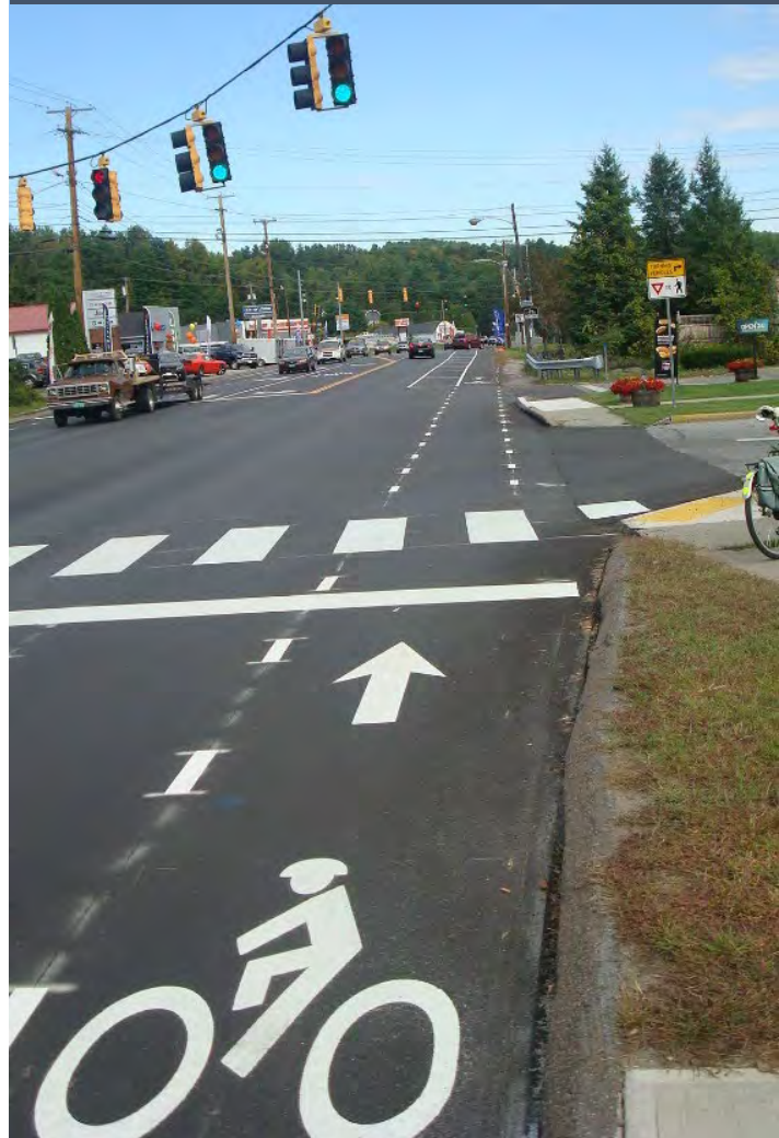
Figure 14. A standard block pattern crosswalk and bike lane pavement markings are shown as part of the Barre-Montpelier Road Diet project in Berlin.
