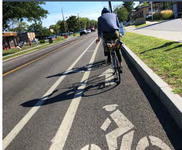
Figure 9. Buffered bike lane in Burlington.
