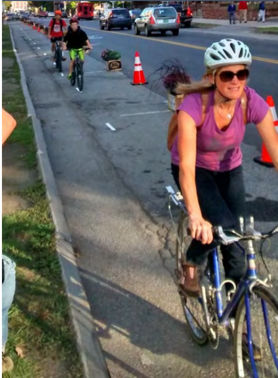
Figure 7. Demonstration bike lane in Montpelier on Class 1 Town Highway. Note that planter boxes are NOT allowed in Vermont State Highway Right of Way.
