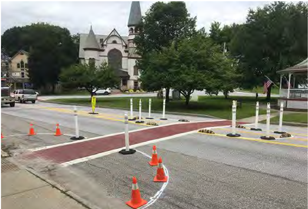
Pictured: Local Motion-assisted demonstration bulb out and pedestrian island on locally managed road in Ludlow, 2021.
