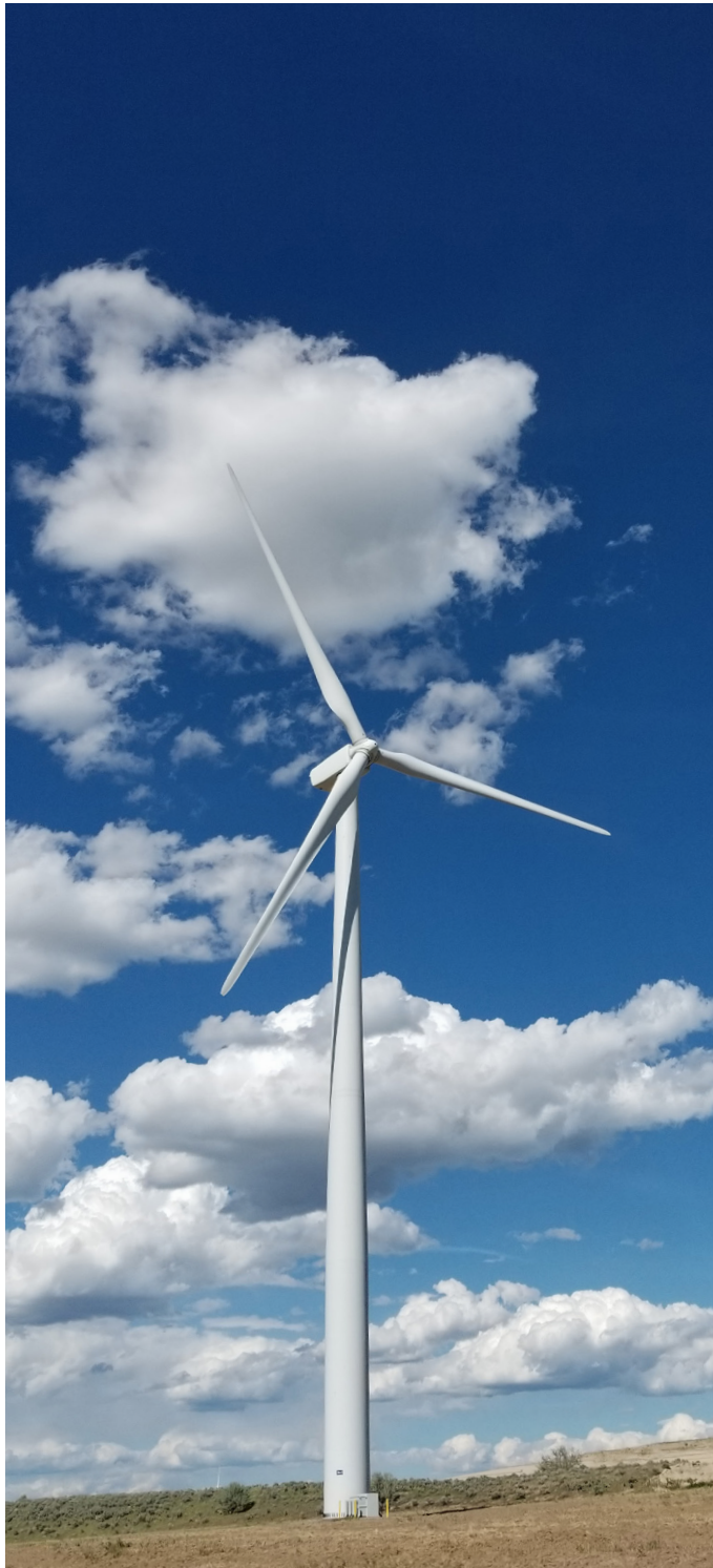
GE 1.6MW wind turbine east of Idaho Falls, ID
