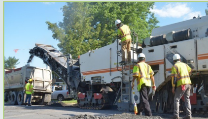
Typical milling operation
