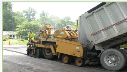
Typical hot mix asphalt paving operation
