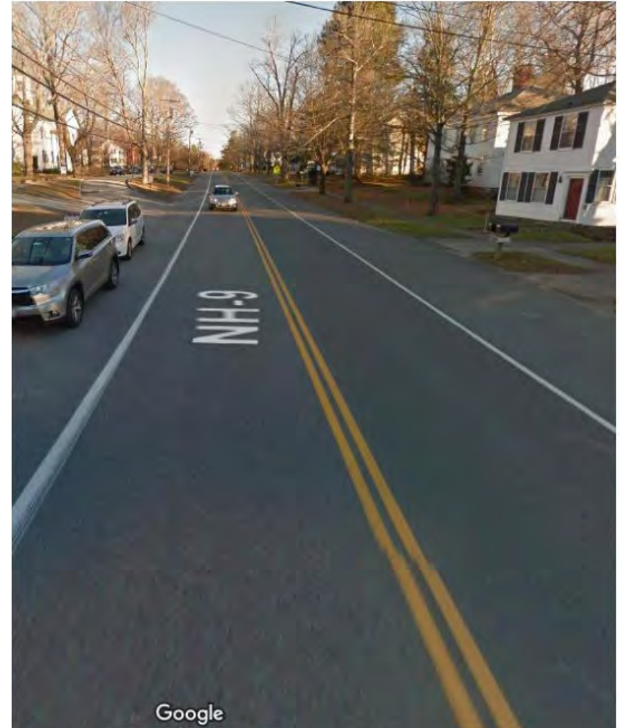
A 10-ft lane installed in Hopkinton, NH
