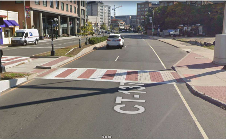
Exhibit 28: Example of decorative crosswalk with continental marked crosswalk in Stamford, CT. (Source: Google Maps Streetview)
