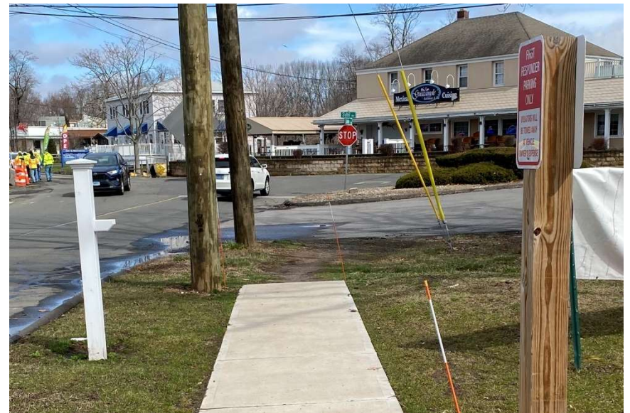
Exhibit 20: No connection to sidewalk at firehouse
