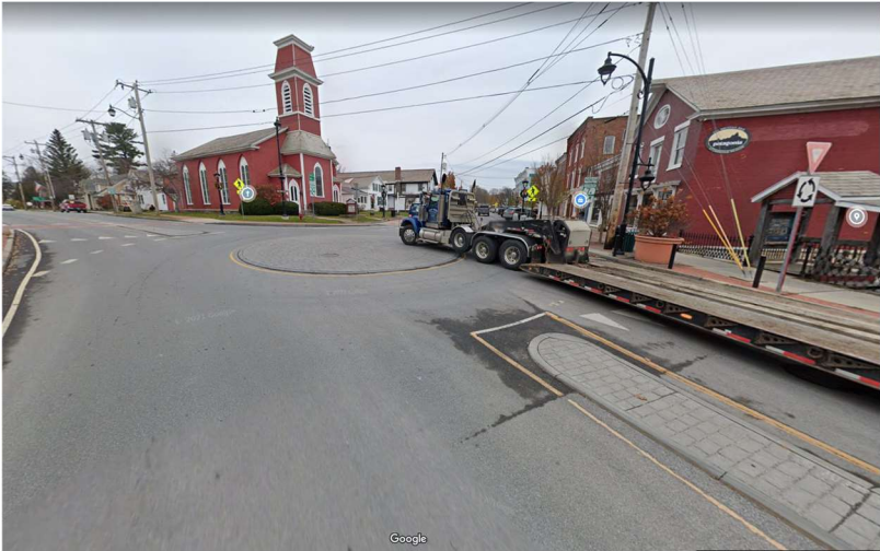
Exhibit 30: Example of a mini-roundabout in Manchester, VT with a diameter of 65-feet. Note the decorative, mountable center island to allow large vehicle movements. (Source: Google Maps Streetview)
