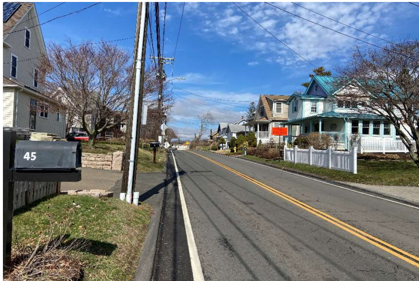
Exhibit 19: Utility poles on Sybil Avenue
