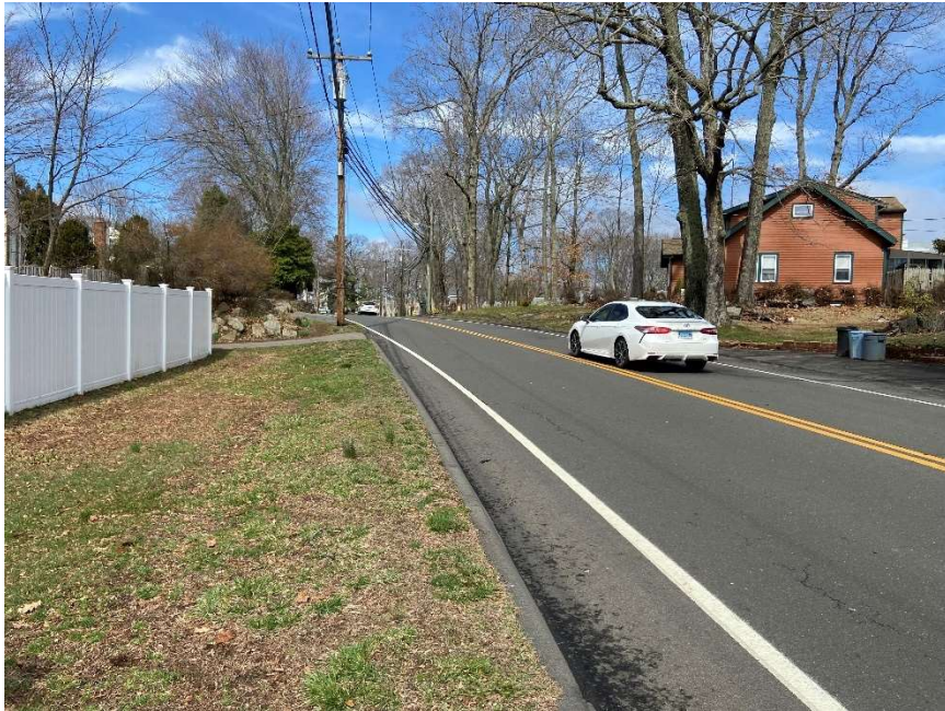
Exhibit 22: View of Route 146 looking north from Block Island Road. Note the vertical grade and reverse curve obstructing sight lines to the north.
