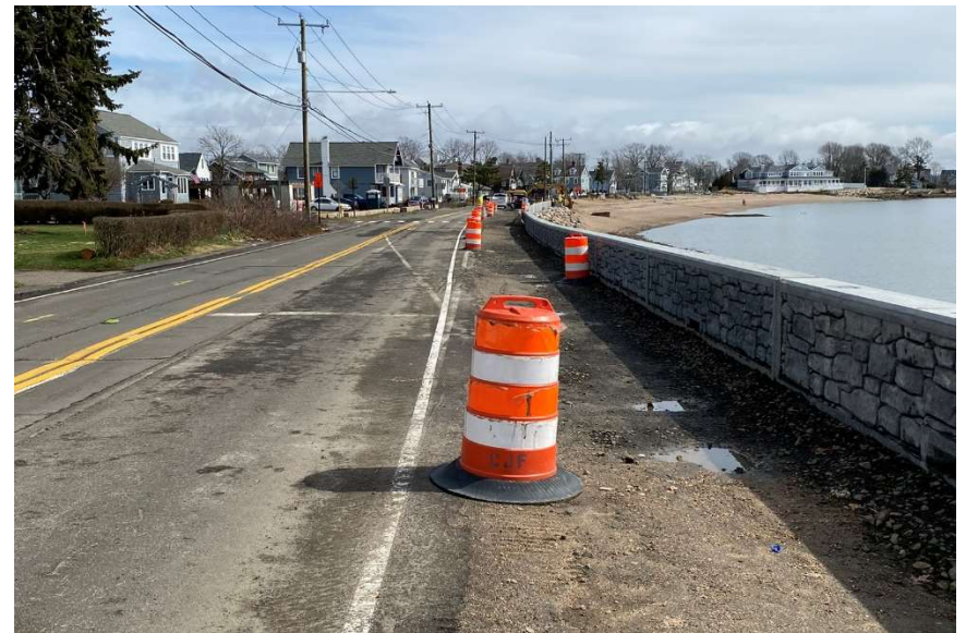
Exhibit 18: Sidewalk construction underway on Limewood Avenue
