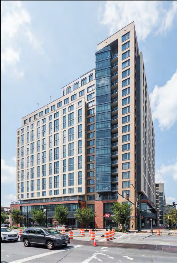
Figure 16. View of 8250 Georgia Avenue in the Ripley District
