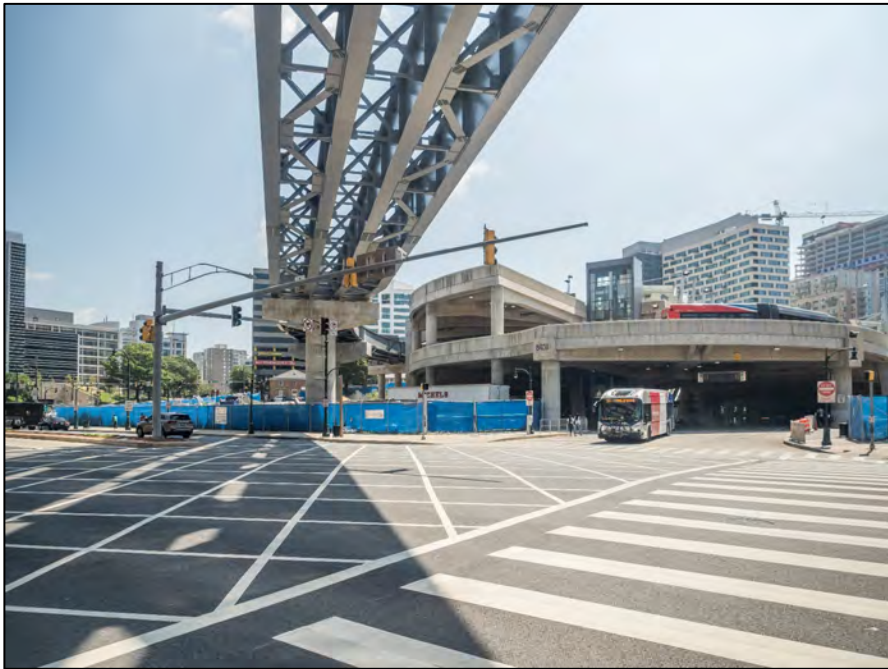
Figure 15. Construction of the Purple Line in the Metro Center District
