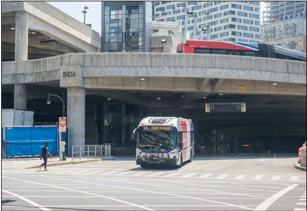
Figure 47. Paul S. Sarbanes Transit Center
