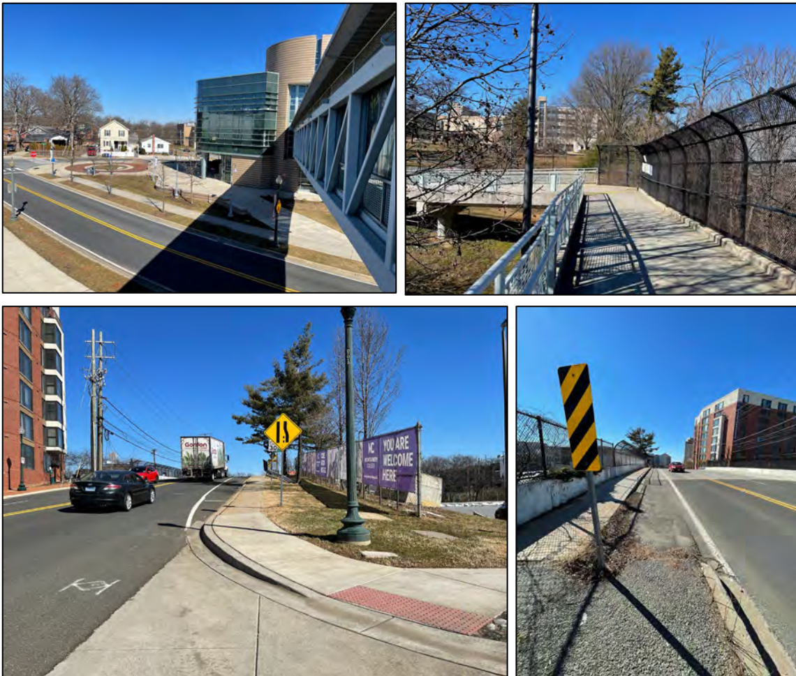
Figure 7. Existing Connections at Montgomery College (Top) and Burlington Avenue (Bottom)
