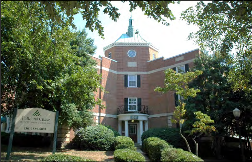
Figure 24. Falkland Chase Apartments
