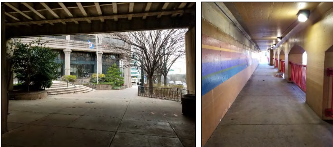
Figure 6. Colesville Avenue Underpass (L); Georgia Avenue Underpass (R)
