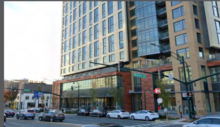
View of 8250 Solaire at Georgia Avenue and Bonifant Street
