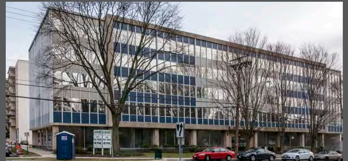
The former Operation Research Institute building will be surveyed to record its architectural significance and its association with the picketing of the office of Carl Freeman by the Action Coordinating Committee to End Segregation in the Suburbs.
