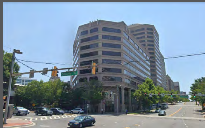
View south on East West Hwy at Colesville Road
