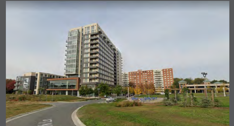
View of the Pearl and large open space
