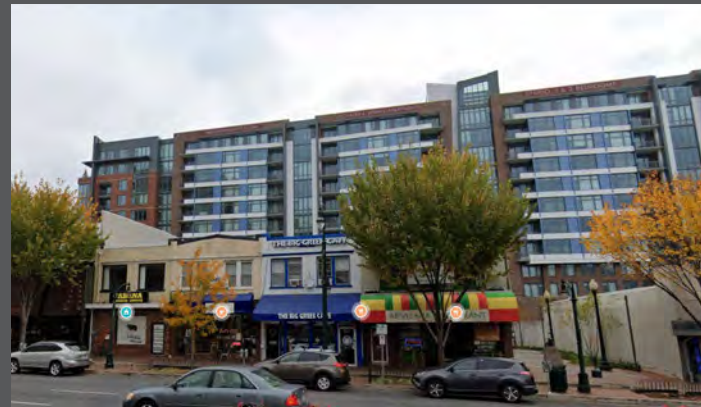
View from Georgia Avenue looking east at Studio Plaza
