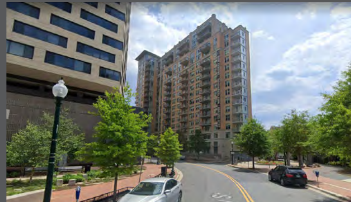
View on Ripley Street Looking north to 1150 Solaire
