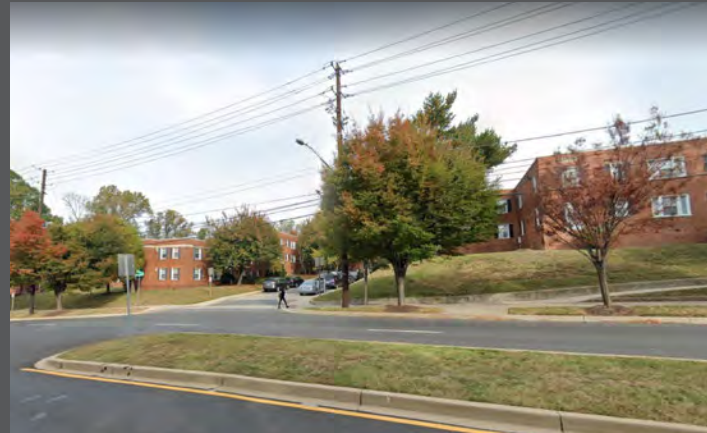
View of Falklands Apartment looking north from E.W. Hwy
