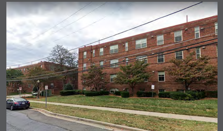
View of Spring Apartments from Eastern Avenue
