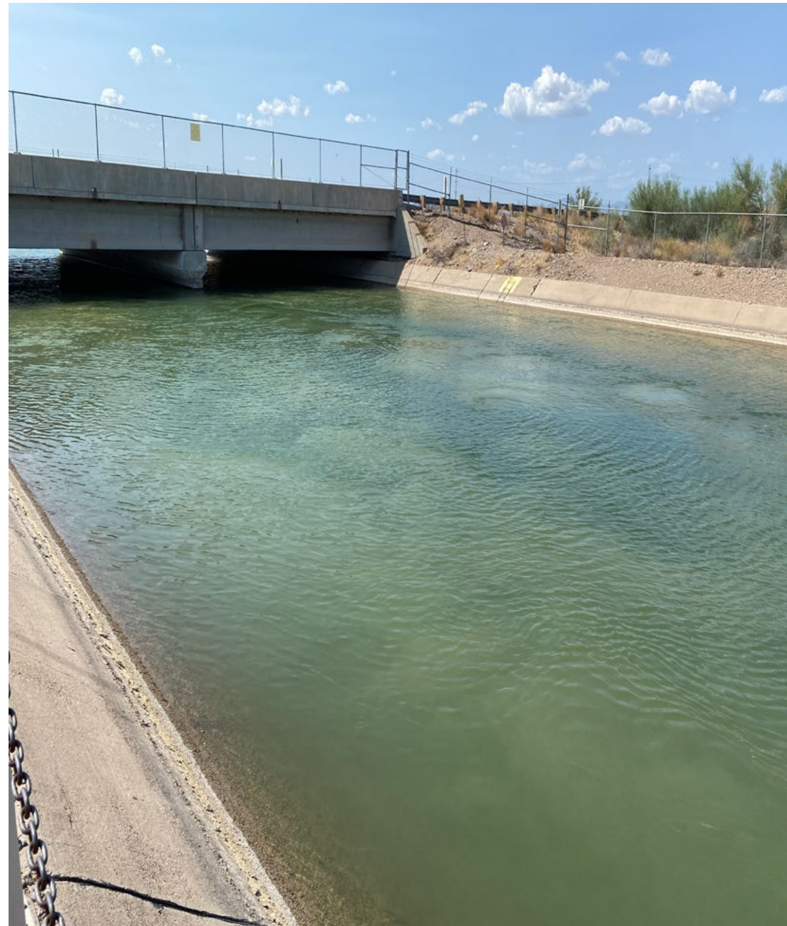
SEDIMENT (TURBIDITY) INCREASES WHEN PUMPS AT HSY ARE ACTIVATED AFTER SUMMER OUTAGE.
