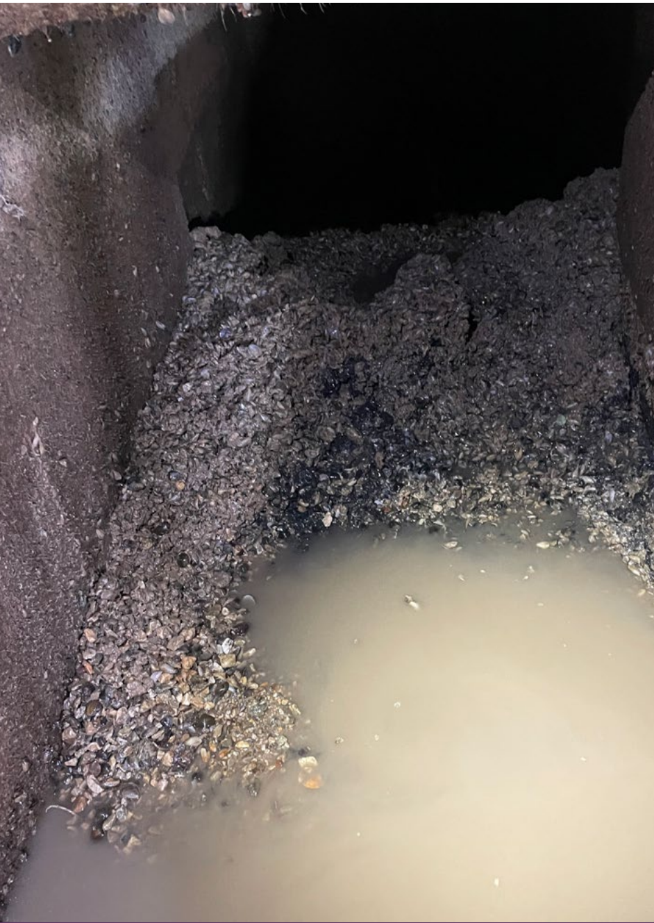
QUAGGA MUSSELS AND CLAMS IN MUD VALVE AT BSH
