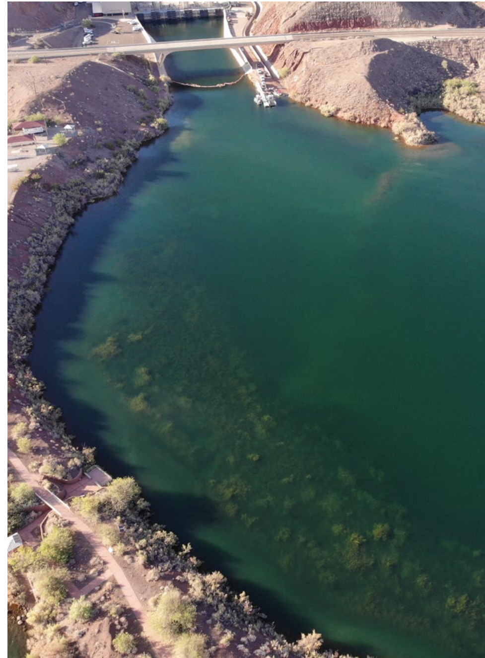
AQUATIC WEED GROWTH WITHIN THE MWP INTAKE CHANNEL IN JUNE 2022
