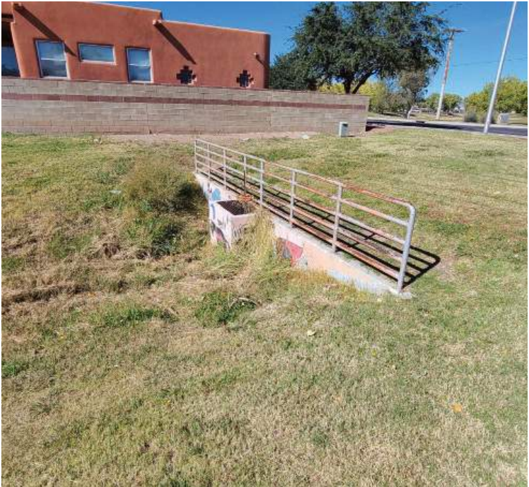
Stormwater outfall at the northwest corner
