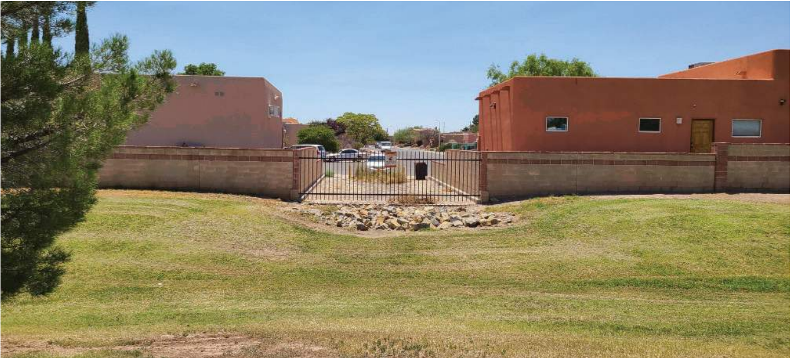
Stormwater outfall from the subdivision to the east
