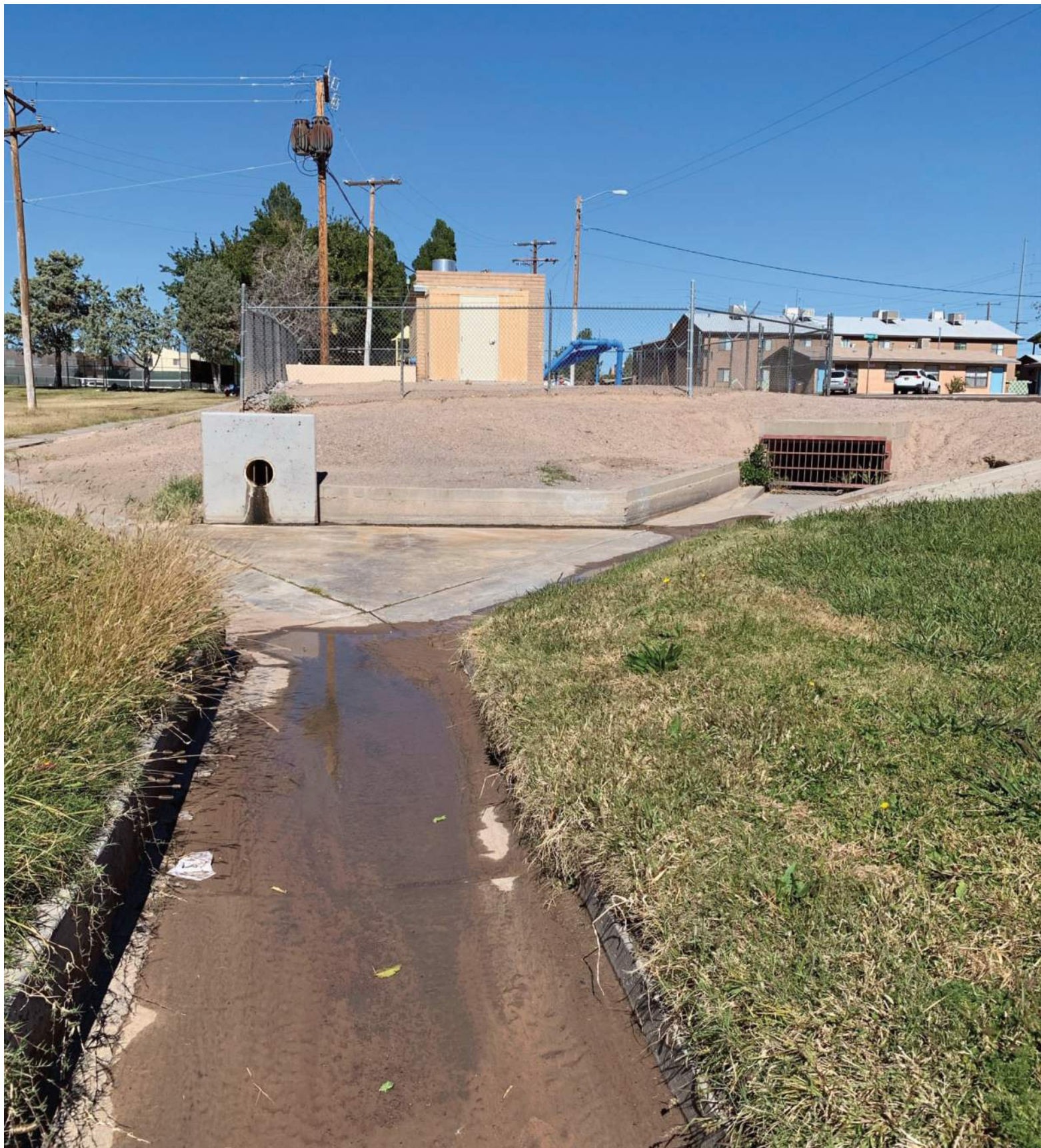
Surface water, subsurface stormwater, and well overflow all discharge to the channel
