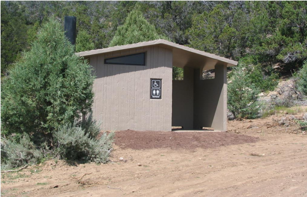
Figure 36: Chamberlain Ranch trailhead pit toilet installed in 2011.
