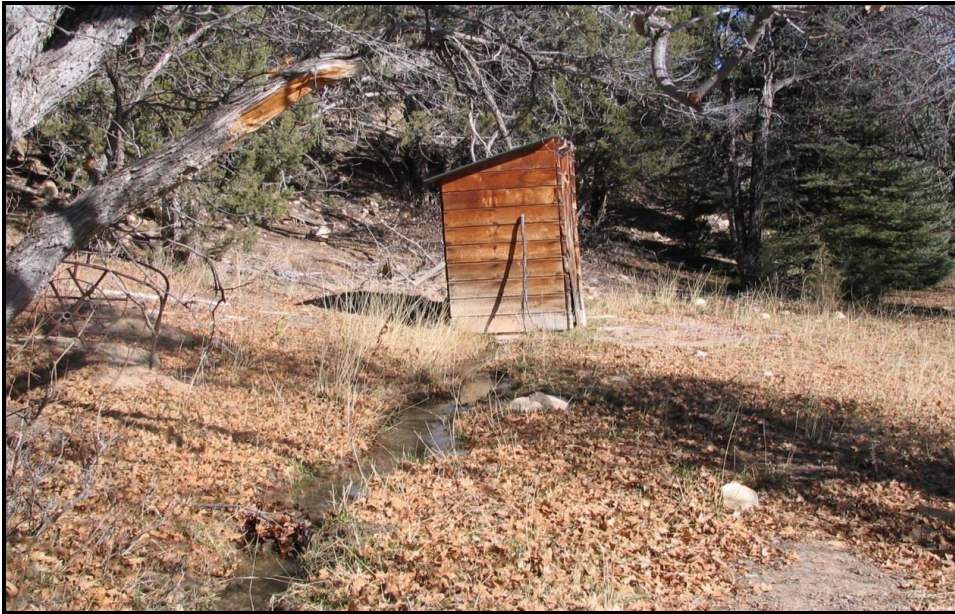
Figure 32: Outhouse constructed over irrigation canal. This structure was removed in 2015.
