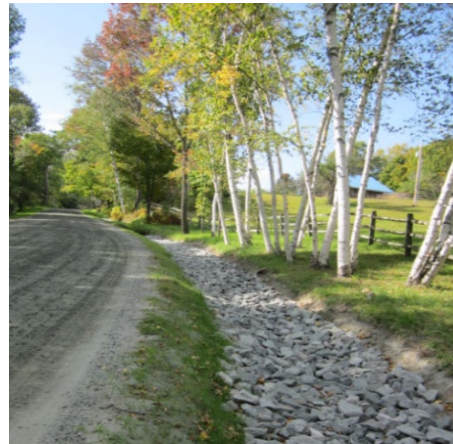
Figure 31. During (left) and after (right) the construction of stone-lined drainage ditch in the Town of West Windsor. Project funding provided by VTrans Better Roads Program. (Source: VTrans)
