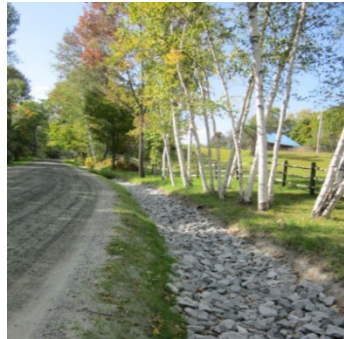
West Windsor drainage ditch improvement funded by Agency of Transportation Better Roads Program
