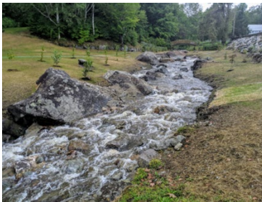
Cold Spring Brook Dam Removal funded by DEC's Clean Water Initiative Program
