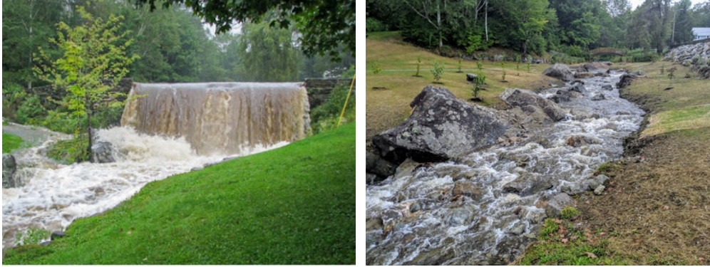
Figure 35. Before (left) and after (right) the removal of the Cold Spring Brook Park dam in the Town of Weston, which restored over 351 linear feet of stream and reconnected 0.2 acres of floodplain. Project funded by a DEC Clean Water Initiative Program grant. (Source: Weston Community Association)
