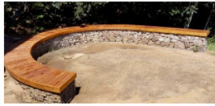
wood-topped gabion baskets
