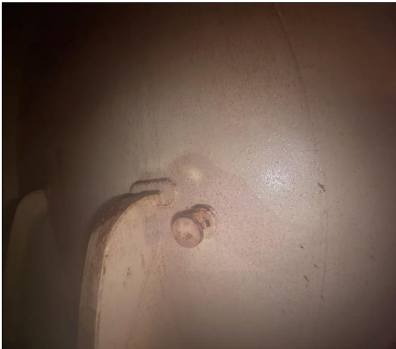
Figure 32. A 3.5" ballast pipe penetration sealed at the outboard bulkhead in A-33F at FR 52-53.
