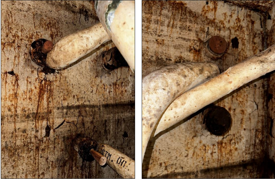
Figure 7. Sealed bulkhead penetrations to tank A-3F. Photographs captured in A-704A.
