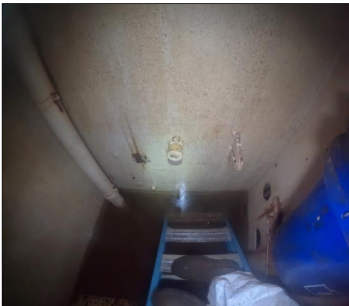
Figure 30. A 2.5" penetration sealed at the inboard bulkhead in A-33F at FR 55-56.
