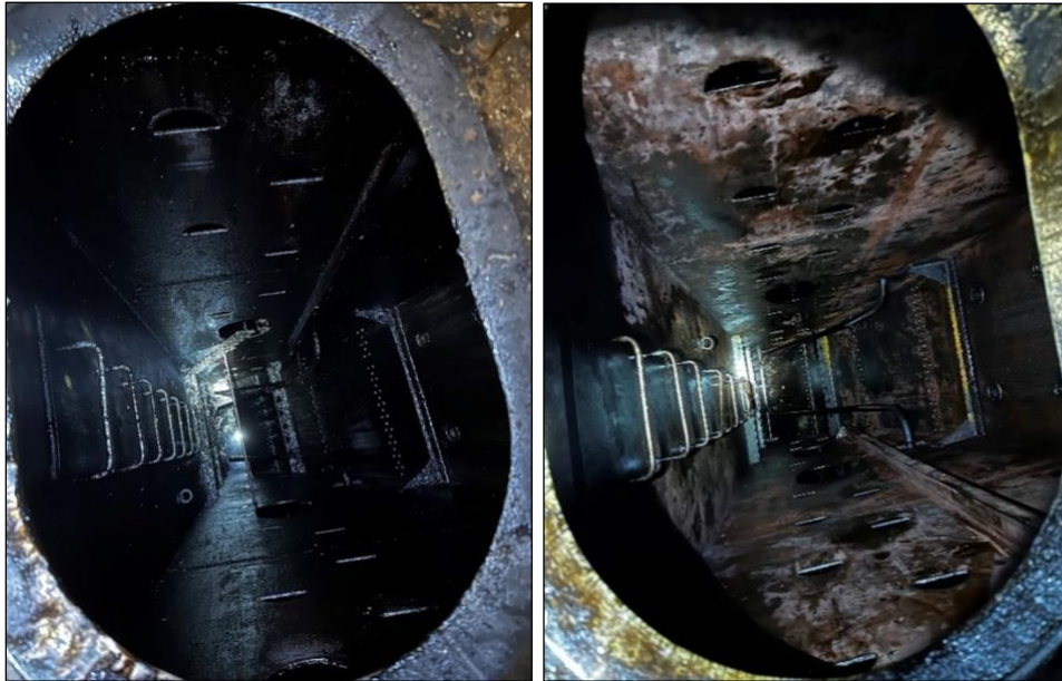
Tank A-62 prior to cleaning
