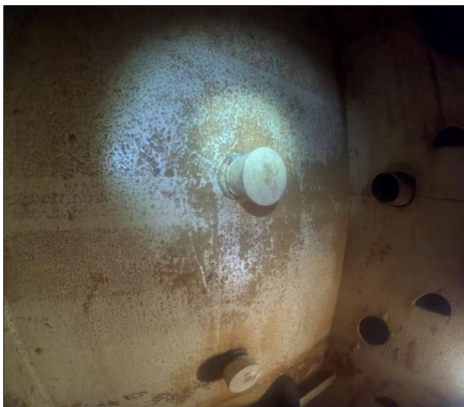
Figure 36. Ballast pipe and fuel oil pipe penetrations sealed at the inboard bulkhead in A-46F. Photograph captured in A-46F.
