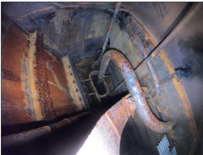
Figure 11. Piping in A-8F prior to removal.
