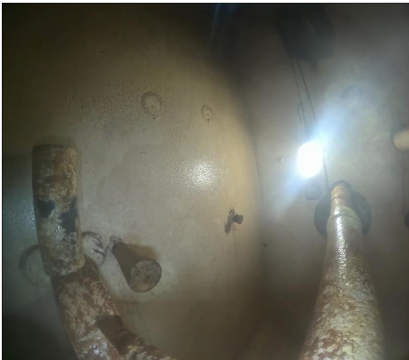
Figure 34. Two 1.5" penetrations sealed at the outboard bulkhead in A-33F at FR 53-54.
