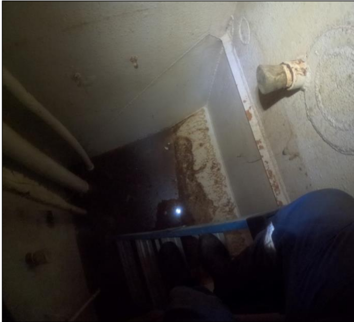
Figure 25. Two 2.5" penetrations sealed at both bulkheads in A-32F at FR 58.
