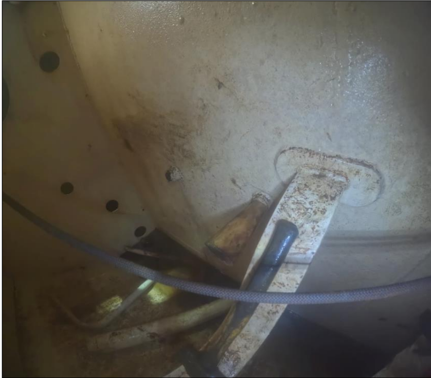
Figure 33. Two 1.5" penetrations sealed at the inboard bulkhead in A-33F at FR 53-54.
