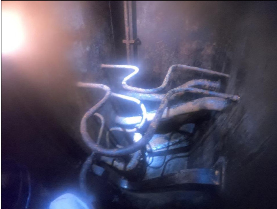
Figure 14. Piping in A-20F prior to removal.
