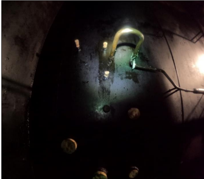
Figure 23. Penetrations sealed at the inboard bulkhead in A-21F.
