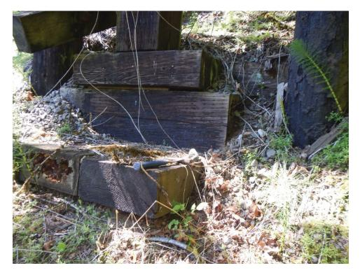
BRIDGE 12 - BENT 11 DECAYED MUD SILL
