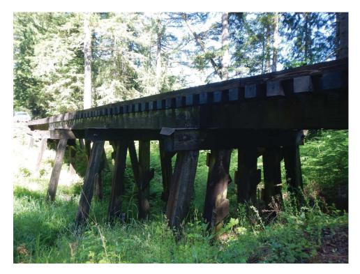
BRIDGE 20 - ELEVATION SHOWING MISSING BRACING
