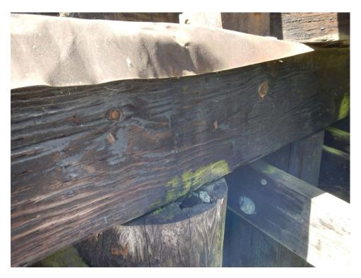
BRIDGE 18 – BENT 1 PILE 5 DECAY AT TOP
