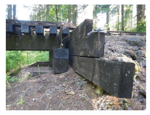
BRIDGE 20 - BENT 7 SHOWING MOVEMENT AND UNDERMINING
