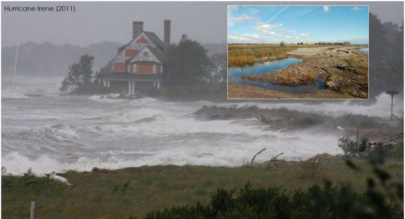
Figure 3. Site Conditions during Tropical Storm Irene (background), Eroded Dune Post-Irene (top right)
