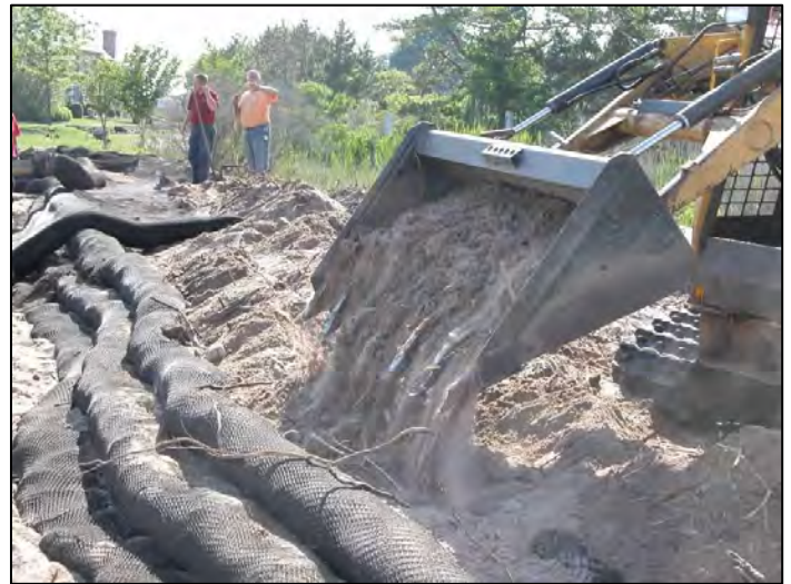
Hepburn Dune Restoration Project 2007: Filtrex tubing filled with sand and mulch
