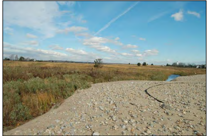
Following Superstorm Sandy, the dune had been leveled, the Filtrexs tubing was lost, and overwash sediment was deposited in the marsh
