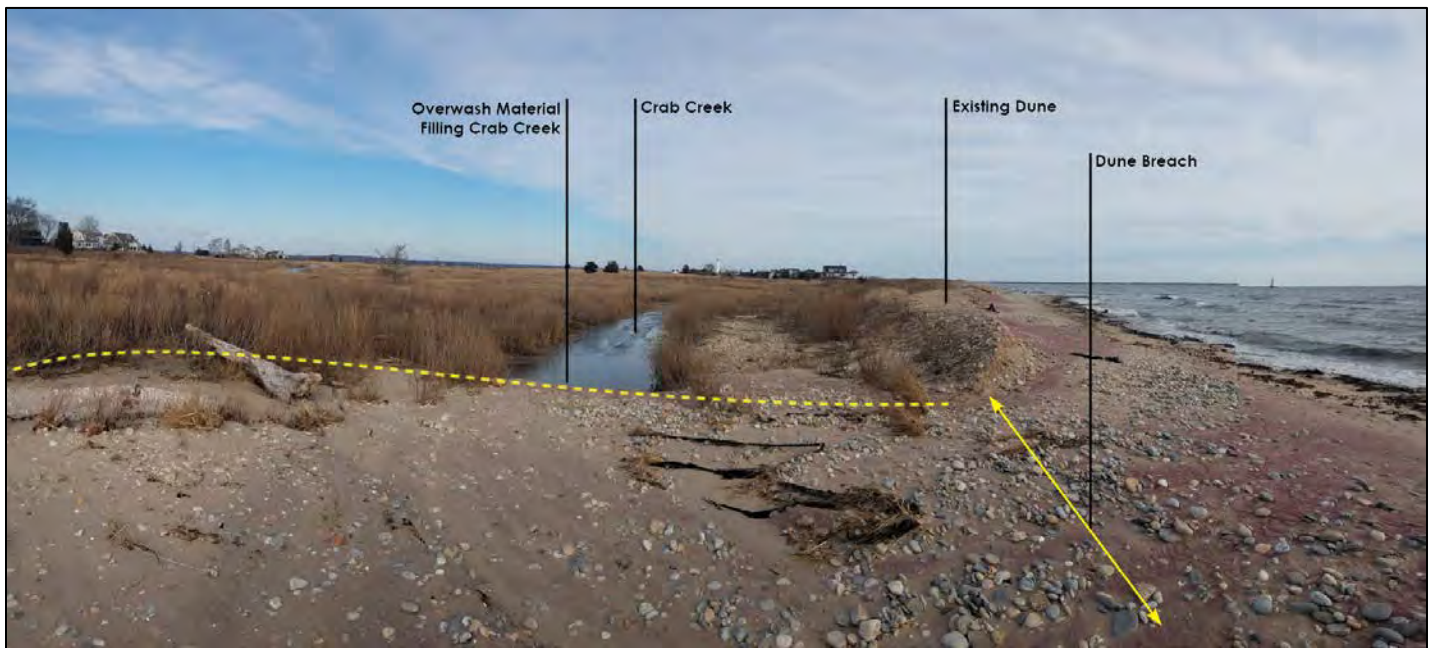
Figure 2: Winter 2019 Dune Breach and Overwash Impacting Crab Creek
