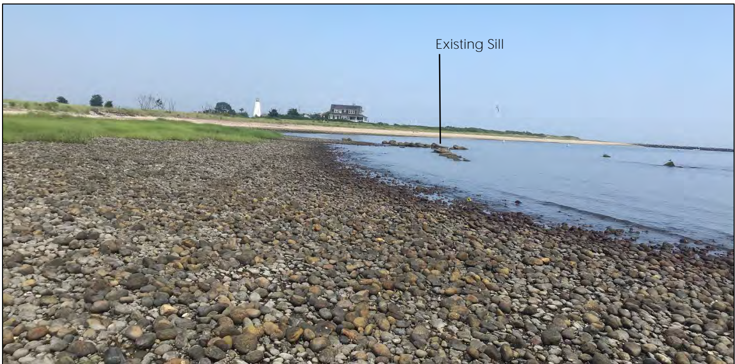
Figure 7 Natural or manmade line of boulders, acting as a sill, contributing to existing marsh growth
