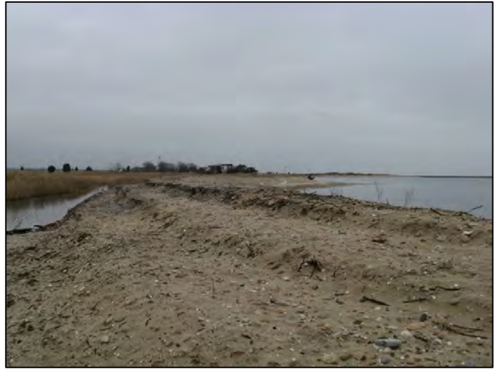
Hepburn Dune Restoration Project Fall 2007: Filtrexx tubing covered with sand
