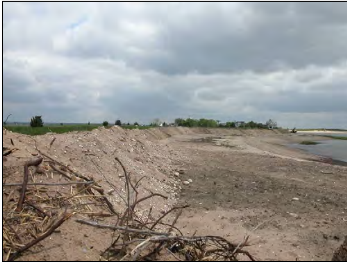
Hepburn Dune Restoration Project Fall 2007: Filtrexx tubing covered with sand
