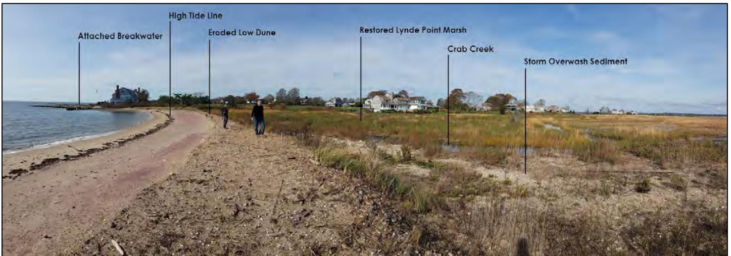
Figure 3 Existing dune and marsh conditions pre-2019 dune breach (looking west at mid tide)
