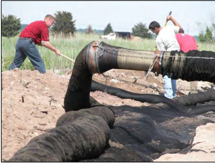
Hepburn Dune Restoration Project 2007: Filtrex tubing filled with sand and mulch
