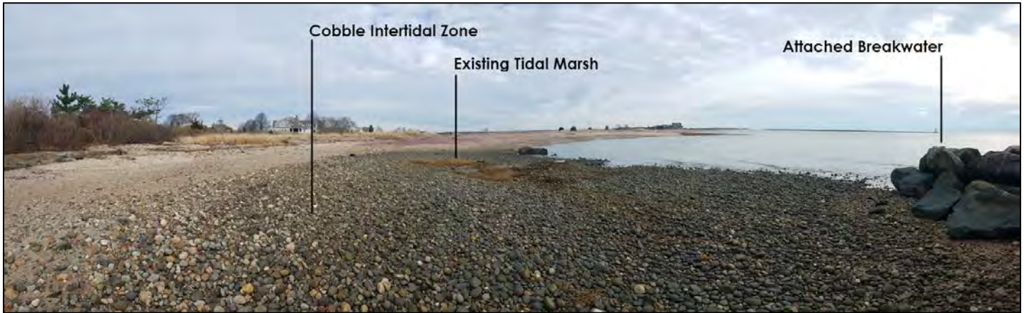
Figure 4 Existing shoreline conditions at west end of site (looking northeast at low tide)
