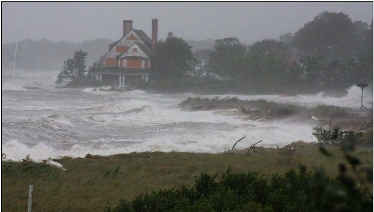
Hurricane Irene (shown) in 2011 and Superstorm Sandy in 2012 caused extensive damage to the dune restoration project
