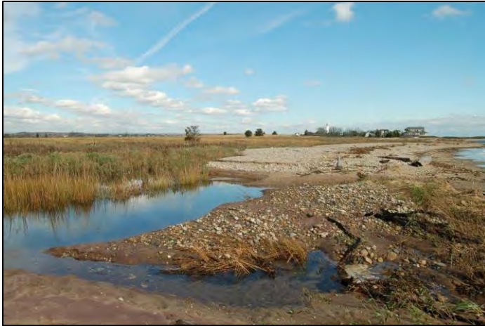
Following Superstorm Sandy, the dune had been leveled, the Filtrexs tubing was lost, and overwash sediment was deposited in the marsh
