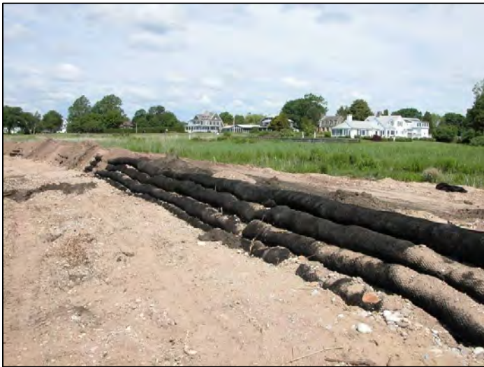
Hepburn Dune Restoration Project 2007: Filtrex tubing filled with sand and mulch
