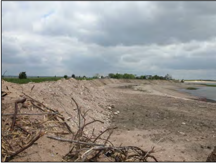
Hepburn Dune Restoration Project Fall 2007: Filtrexx tubing covered with sand
