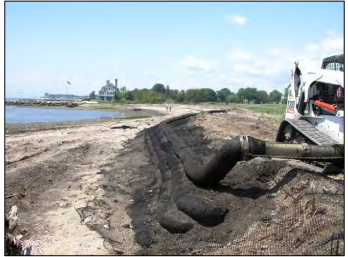
Hepburn Dune Restoration Project 2007: Filtrex tubing filled with sand and mulch
