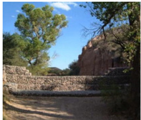
Figure 2. Photographs of rock detention structures (RDS) in riparian areas in the Madrean Ecoregion, including a.) a one-rock dam (Tosline et al., 2020), b.) a check dam (Norman et al., 2015), and c.) a gabion (Norman et al., 2014).
