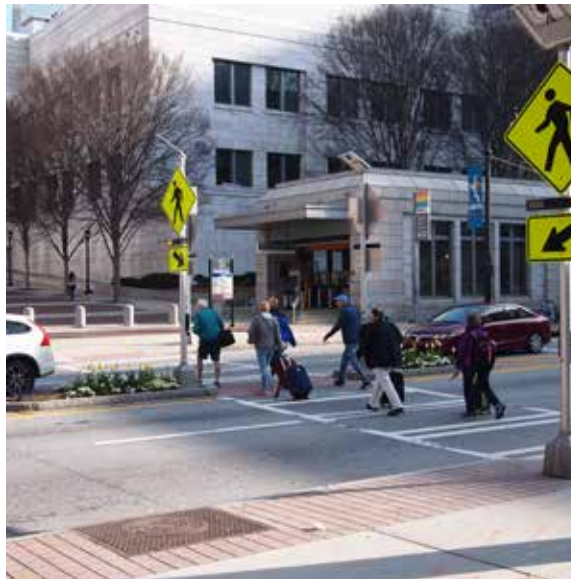
Marked crosswalk with RRFB and refuge island.
