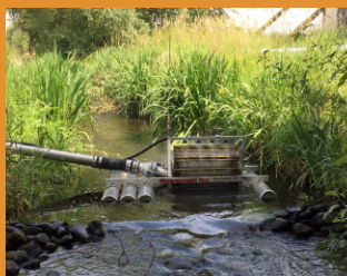
Installing fish-friendly screens on irrigation intakes.
