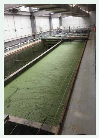
Photo: Michele Burford Harvesting *Microcystis* using dissolved air flotation water treatment technology.
