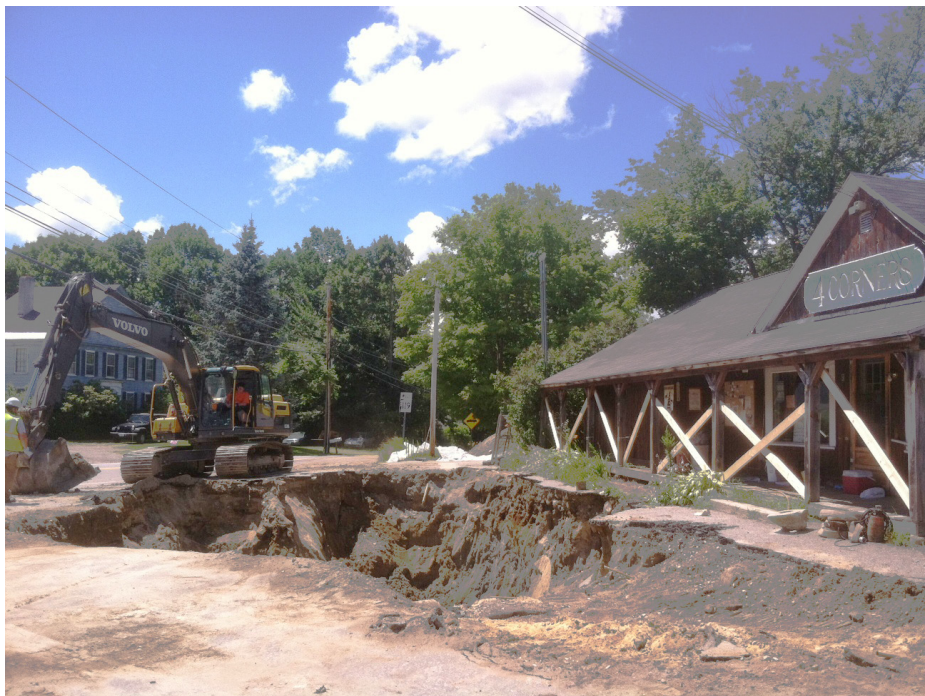
Figure 1. July 2014 contaminated soil excavation at the Richmond Four Corners Store.
