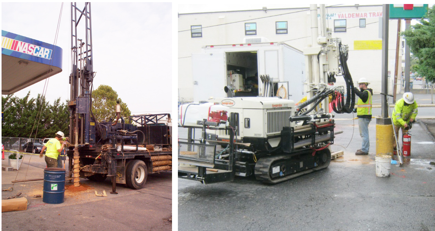
Figure 1. Hollow stem auger (HSA) vs. MIPS and LIF with direct push. Note the waste drum for the HSA rig and the bucket for the direct push—a significantly different amount of waste.
