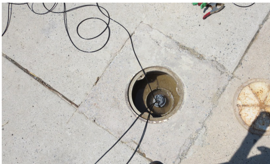
Figure 2. A multi-level (“CMT”) bedrock monitoring well with multiple groundwater elevation gauges. A single well gains the same data as five separate wells at multiple elevations.
