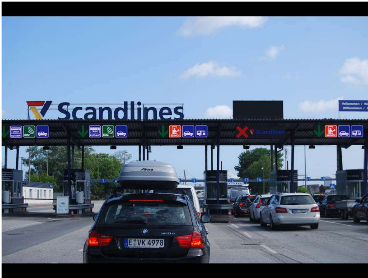
Figure 4 - Entrance gates to the Puttgarden terminal where fares are collected. The two gates on the left are being used for electronic fare collection.
