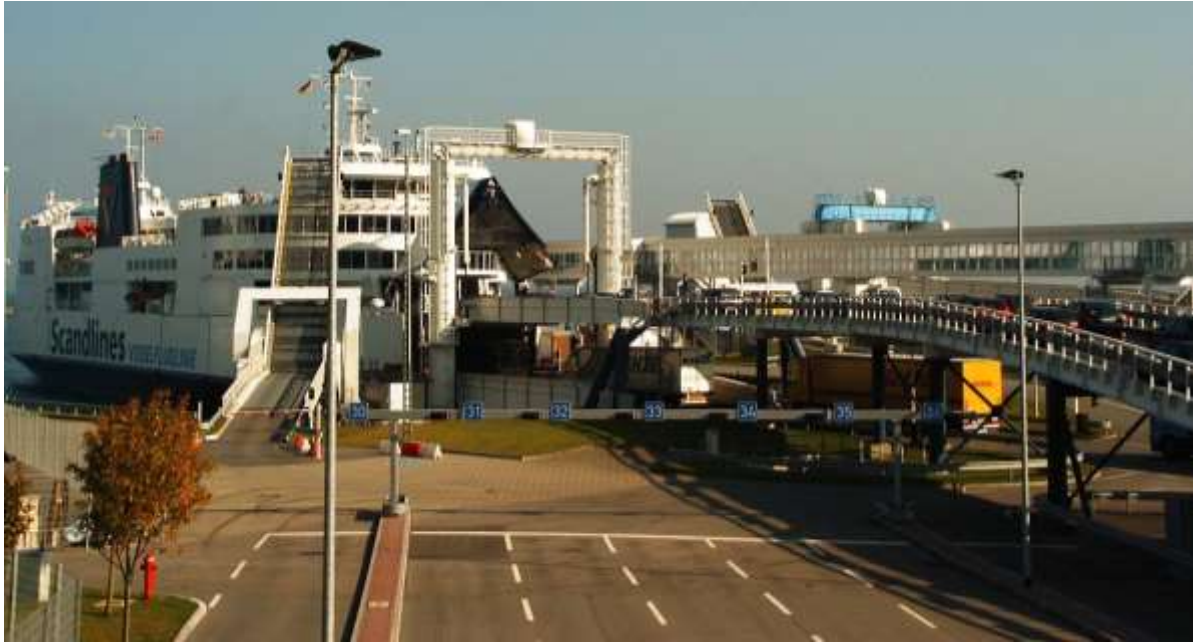
Figure 5 - Ferry vessel docked at Puttgarden. Loading/unloading ramps and roads visible with staging area in the foreground
